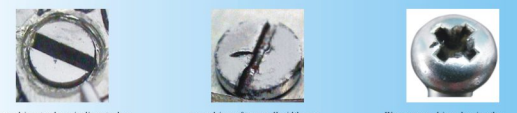
screwdriver too large in diameter has been used. A corner of the screwdriver has gouged out the plate leaving irreparable damage. screwdriver of too small width was used, leaving the screw head burred up and unusable. Wrong screw driver, leaving the screw head burred up (using a Pozidriv screw driver on a Phillips head)
